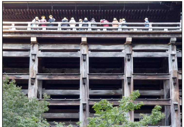
Supports under the main building at Kiyomizu Temple. All wood, no nails!
